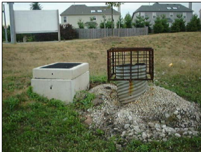
FIGURE 5-8 Sediment filter left in place after construction. SOURCE: Robert Traver, Villanova University.
