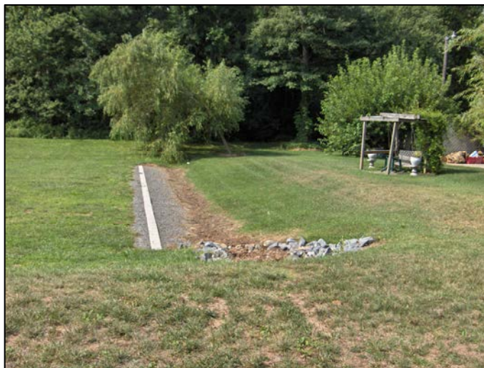
FIGURE 5-11 Level spreader. SOURCE: Robert Traver, Villanova University.
