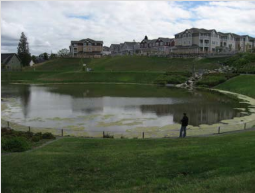
FIGURE 5-58 Natural drainage system methods have been applied to a 34-block, 1,600-unit mixed-income housing redevelopment project called High Point. Shown on top, vegetated swales, porous concrete sidewalks, and frontyard rain gardens convey and treat stormwater on-site. Below is the detention pond for the development. SOURCE: top, William Wenk, Wenk Associates, and bottom, Laura Ehlers, National Research Council.
