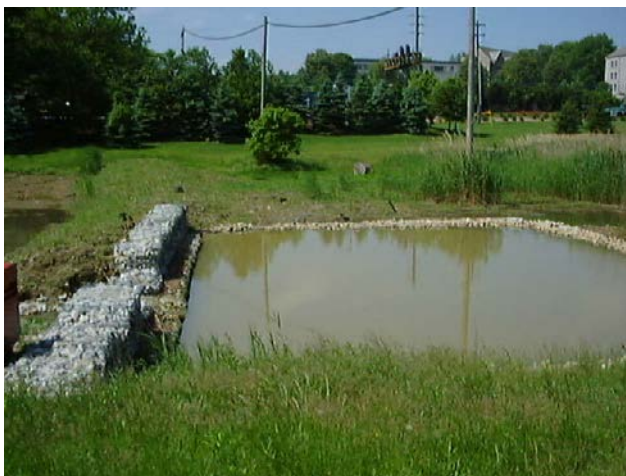
FIGURE 5-44 Villanova University sediment forebay. SOURCE: Reprinted, with permission, from VUSP. Copyright by VUSP.
