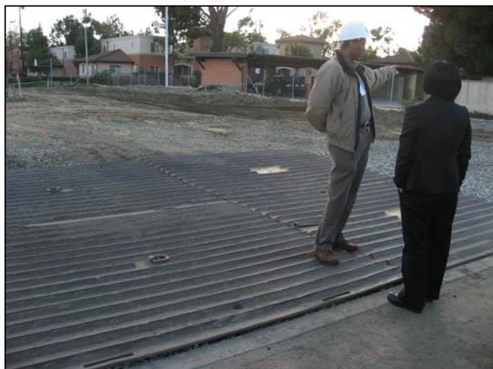
FIGURE 5-10 Rumble strips to remove dirt from vehicle tires. SOURCE: Laura Ehlers, National Research Council.
