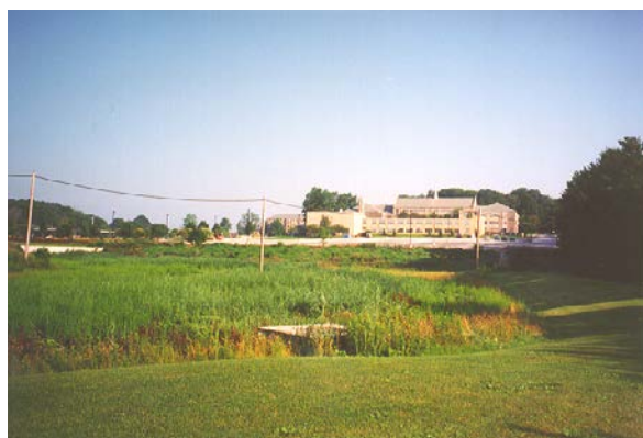
FIGURE 5-41 Retrofitted stormwater wetland at Villanova University. SOURCE: Reprinted, with permission, from VUSP. Copyright by VUSP.
