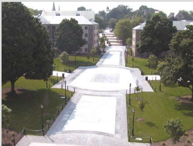
FIGURE 5-33 Villanova University pervious concrete retrofit site. SOURCE: Reprinted, with permission, from VUSP. Copyright by VUSP.
