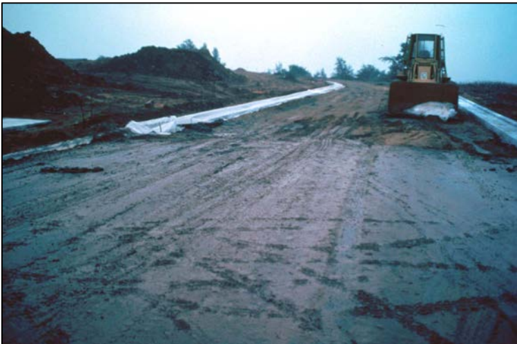
FIGURE 3-35 Construction site in early spring after snowmelt showing extensive sediment transport. SOURCE: Roger Bannerman, Wisconsin Department of Natural Resources.
