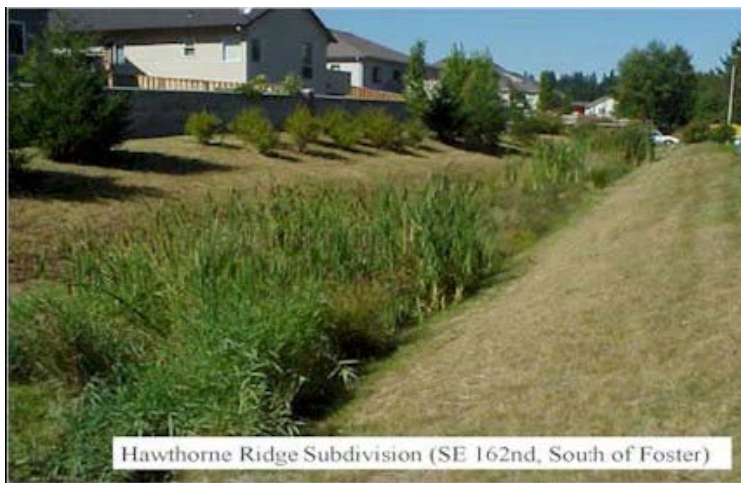
FIGURE 5-16 Vegetated swale. SOURCE: PaDEP (2006).
