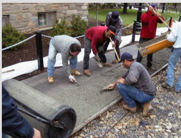
FIGURE 5-34 Infiltration bed under construction. Pervious concrete has functionality and workability similar to that of regular concrete. However, the pervious concrete mix lacks the sand and other fine particles found in regular concrete. This creates a significant amount of void space which allows water to flow relatively unobstructed through the concrete. This site was the first attempt at creating a pervious concrete SCM in the area, and there were construction and material problems. Since that time the industry has matured, and a second site on campus constructed in 2007 has not had any significant difficulties. SOURCE: Reprinted, with permission, from VUSP. Copyright by VUSP.
