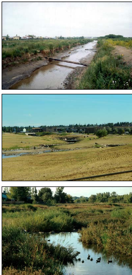
FIGURE 5-48 Three photographs illustrate stream rehabilitation in Denver. The top picture is a creek that has eroded in its bed due to urbanization. The middle picture shows a portion of the stabilized creek immediately after construction. Check structures, which keep the creek from cutting its bed, are visible in the middle distance. The bottom image shows the creek just upstream of one of the check structures two years after stabilization. The thickets of willows established themselves naturally. The only revegetation performed was to seed the area for erosion control. SOURCE: Courtesy of Wenk Associates.
