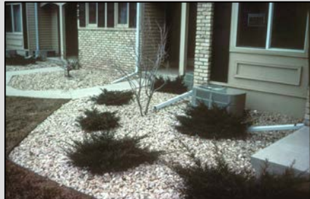
A disconnected roof drain (drains to pervious area)
