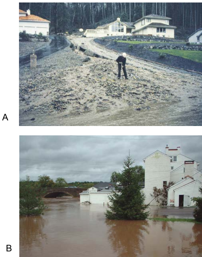
FIGURE 1-6 (A) New residential construction in the path of episodic stream discharge (Issaquah, Washington); (B) recent flooding of an 18 th -century tavern in Collegeville, Pennsylvania following a storm event in an upstream developing watershed. SOURCES: Top, Derek Booth, Stillwater Sciences, Inc., and bottom, Robert Traver, Villanova University.
