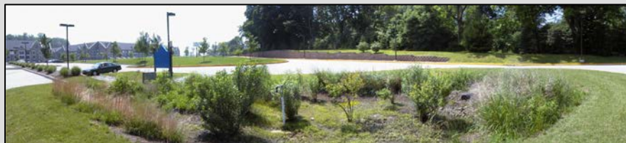
FIGURE 5-21 Villanova Bioinfiltration Traffic Island SCM. SOURCE: Reprinted, with permission, from VUSP. Copyright by Villanova Urban Stormwater Partnership.
