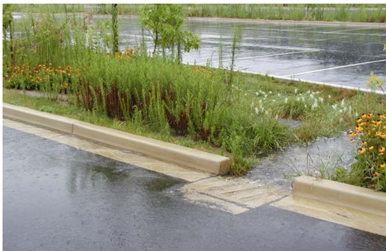
FIGURE 5-17 Bioretention during a storm event at the University of Maryland. SOURCE: Reprinted, with permission, from Davis et al. (2008). Copyright 2008 by the American Society of Civil Engineers.
