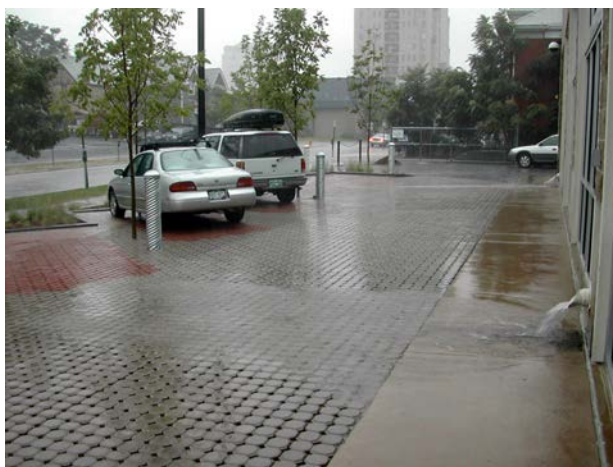
FIGURE 5-32 A small office building conversion at the edge of downtown Denver included the replacement of a portion of the site's parking with modular block porous pavement underlain by an 18-inch layer of crushed rock. Rainfall on the porous pavement and roof runoff for most storm events are contained in the reservoir created by the crushed rock. The pavement infiltrates runoff from most storm events for one-third of the impervious area on the half-acre site. SOURCE: Courtesy of Wenk Associates.
