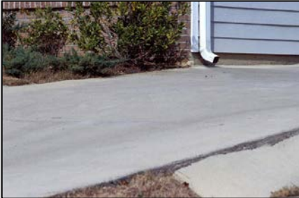
A directly connected roof drain
