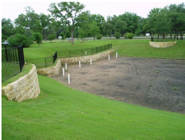
FIGURE 5-45 Austin sand filter. SOURCE: Robert Traver, Villanova University.
