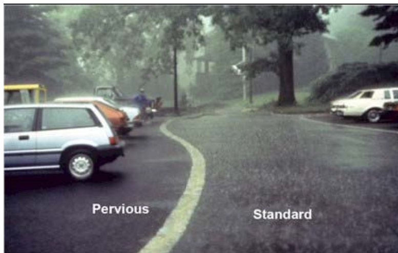
FIGURE 5-29 Porous asphalt. SOURCE: PaDEP (2006).
