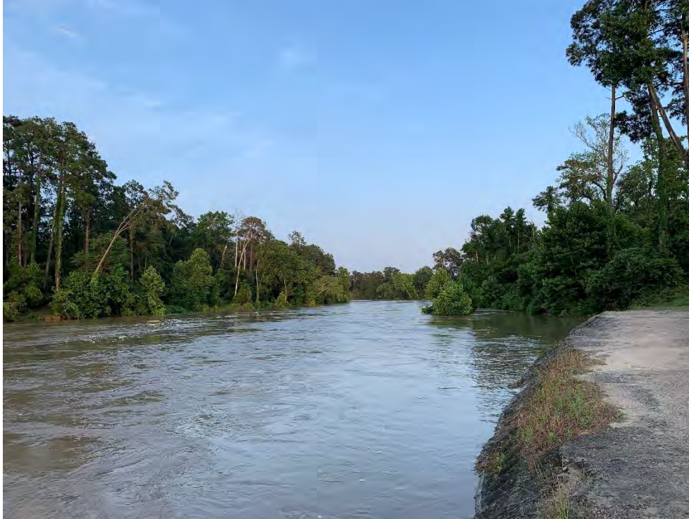
Figure 2-3. Spring Creek channel downstream of I-45.
