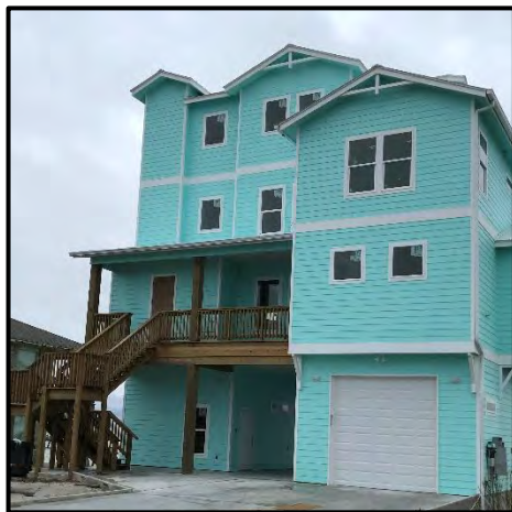
Above: This well built home in the community of Copano Village in Aransas County, TX survived Hurricane Harvey in 2017.
