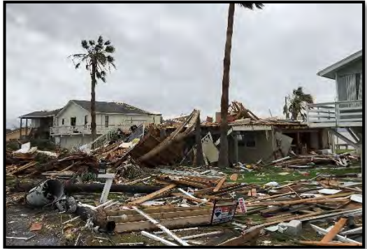
Above: Damage to the community of Copano Village in Aransas County, TX in the wake of Hurricane Harvey in 2017.
