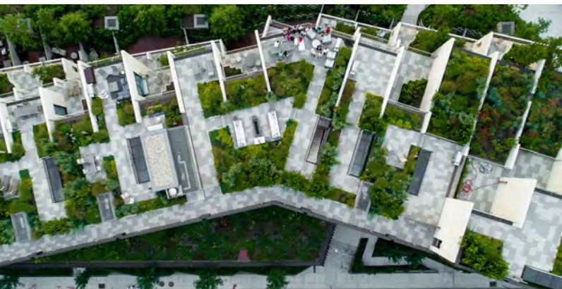
PHOTO: Aerial view of rooftop gardens.
