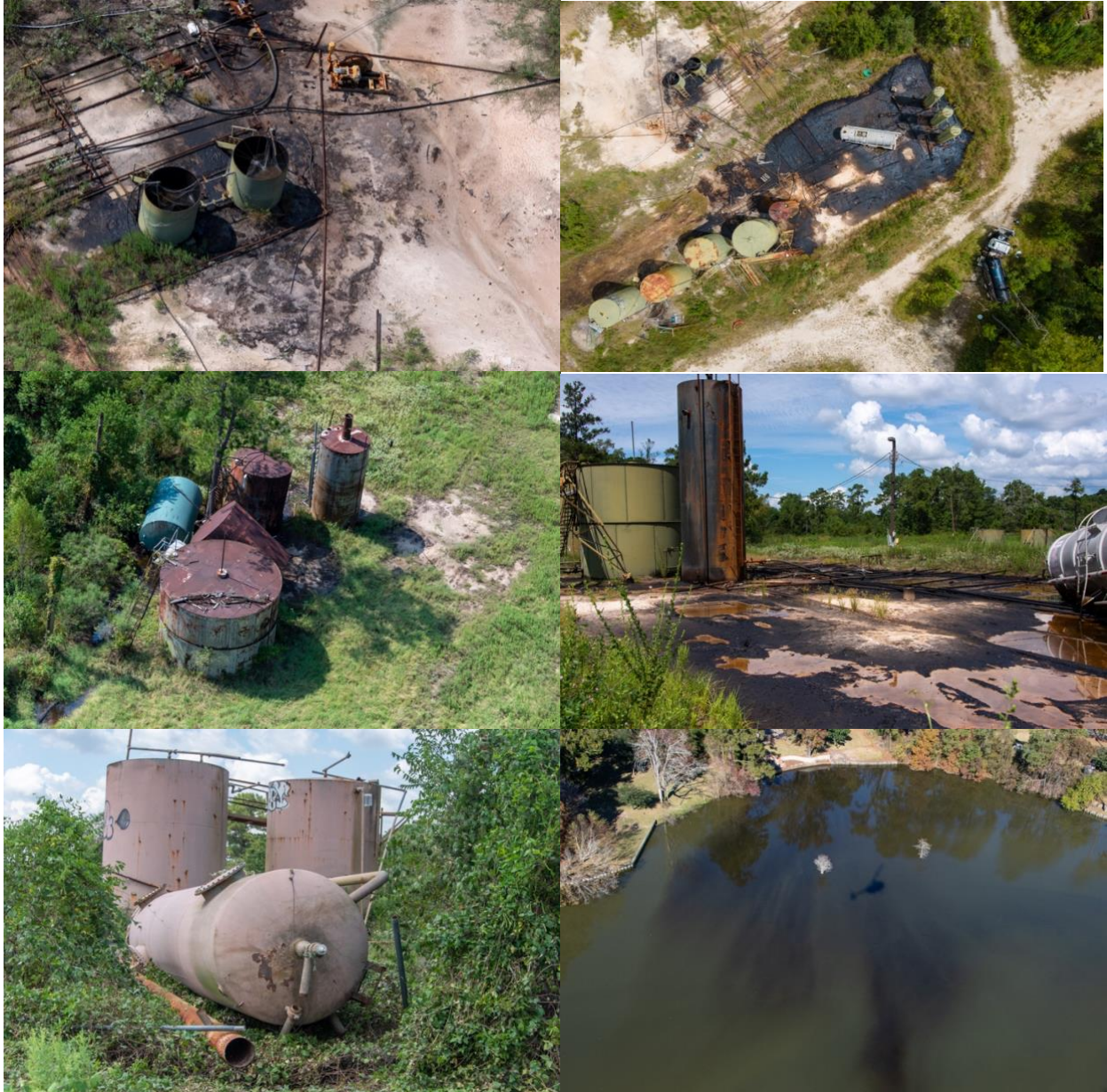
Damage to wells and tanks caused by Harvey that impaired water quality in the West Fork and Lake Houston. All from Forest Cove area within 500 feet of West Fork.
