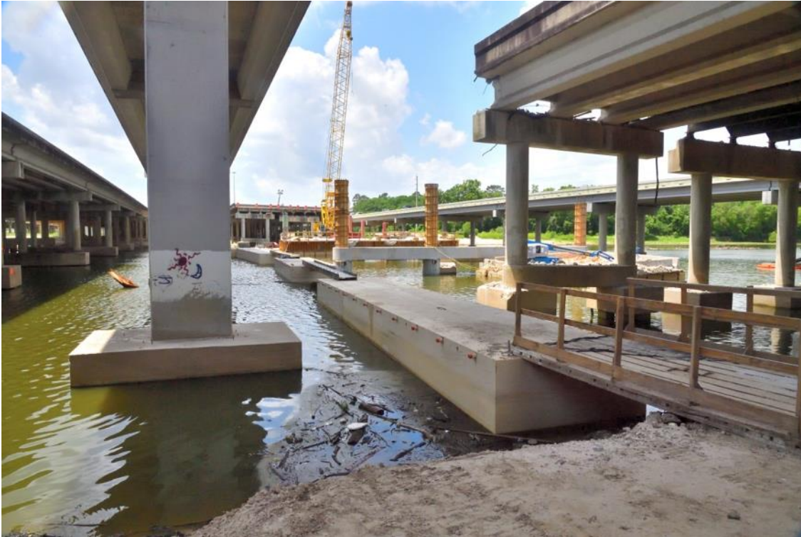
Looking south toward Humble at I-69/West Fork Bridge repairs after Harvey
