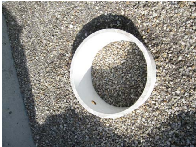
Figure 4: Pipe installed in media
