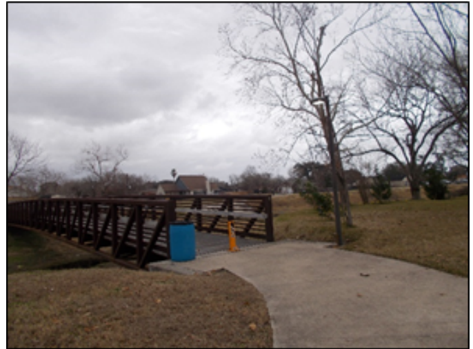
A bridge that crosses over the expanded Lone Tree Creek Channel. Photo by Joyce Price/FEMA
