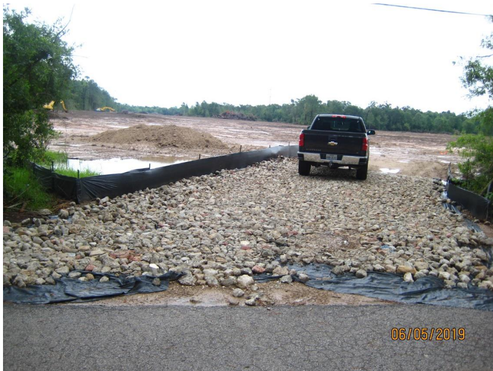
Entrance/Exit has been stabilized with rock; corrective actions completed
