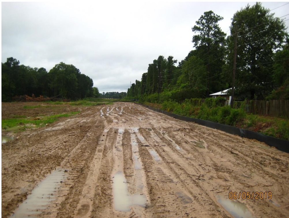
Silt fence installed; corrective actions completed
