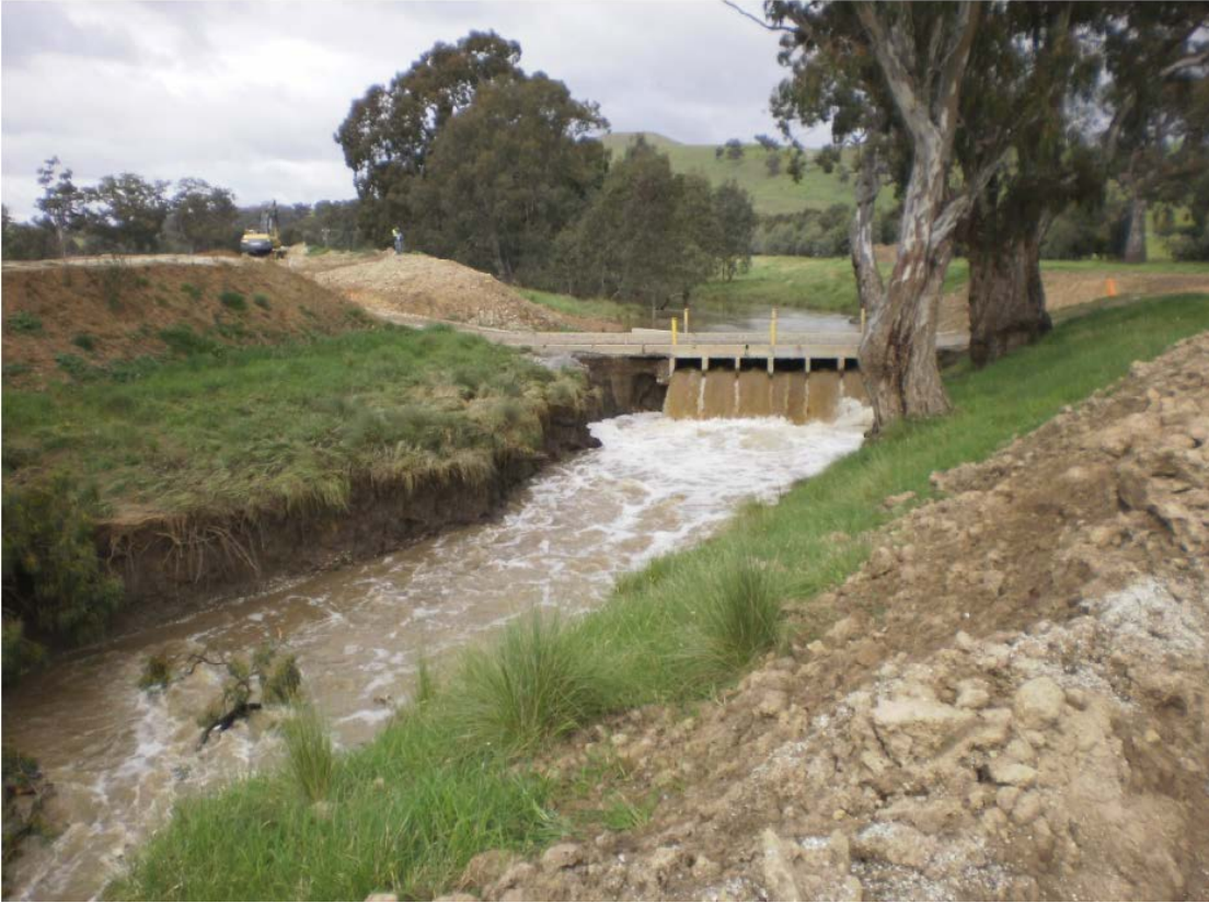
Figure 2. Upstream progressing erosion caused when Island Creek broke into a gravel mine on the Goulburn River floodplain (Craigie, 2012)
