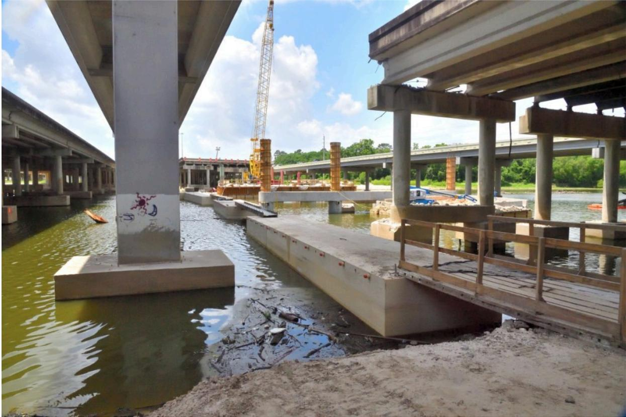
*The southbound lanes of I-69 had to be completely rebuilt after Hurricane Harvey because of scouring that undermined bridge supports and structural integrity. The \$20 million TxDOT project delayed in- and outbound traffic for ten months.*
